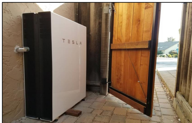
Fig. 19: The Tesla Powerwall is one of the most popular battery storage systems for solar. This relatively small container can supply an average-size house for one day. (Leon, 2018)
