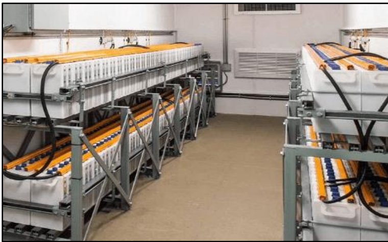
Fig. 18: Lithium Battery Bank. Schroeder, D. (n.d.)
