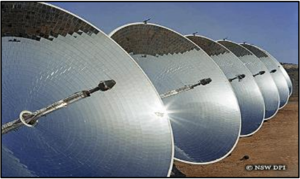
Fig. 24: A Parabolic Solar Dish is a mirrored shape like a satellite antenna. It concentrates light energy on a receiver. - Solar power at White Cliffs (Dpi, 2009)
