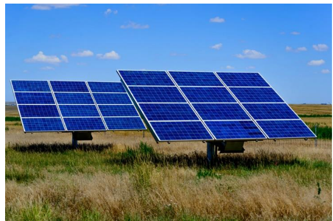
Fig. 16: Ground Mounted Solar Modules in a Field (Darcey)
