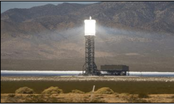
Fig. 23: The Power Tower uses thousands of ground-mounted mirrors that adjust their tracking as the sun moves across the sky. Ivanpah Solar Power Plant (srose15, 2016)
