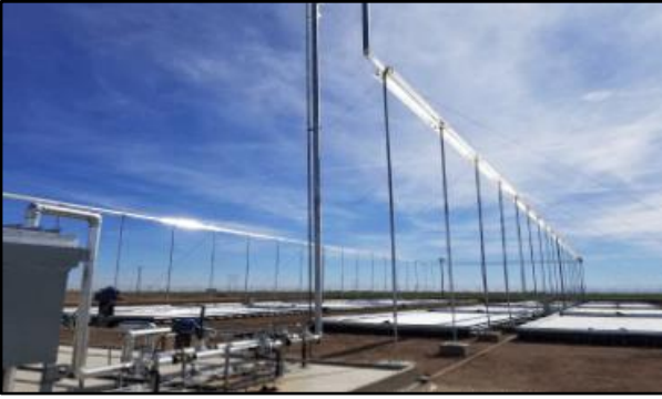
Fig 21: Linear Fresnel. Concentrates light using a series of angled mirrors, generating heat. (Mehos, "Concentrating Solar Power (CSP) Overview", n. d.)
