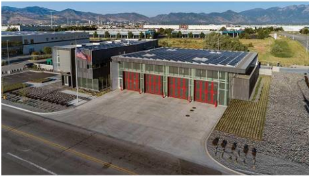
Fig. 3: Salt Lake City's Fire Station 14
