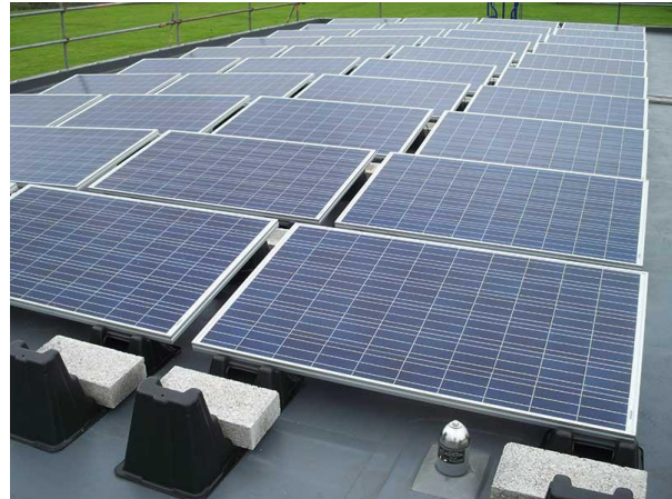
Fig. 11: Ballasted Flat Roof Mounted Solar System (Gupta, 2018)
